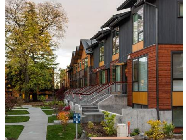
Porches Overlooking Linear Park, Materials Wrapping The Corner Of The Building
