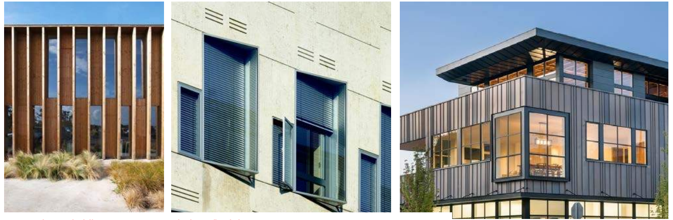
Modulation of windows to create visual interest and depths to the street facade
