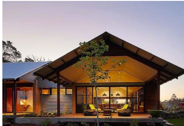
Careful Use of materials and Color Can Create Visual Interest and Breaks Down Scale of the Building
