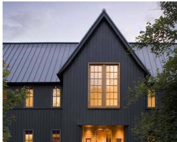
Clean, Uncluttered Roof Line
