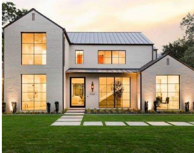
Clean, Uncluttered Roof Line
