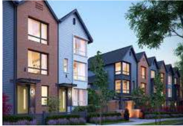
Entry Porches Overlooking Alley
