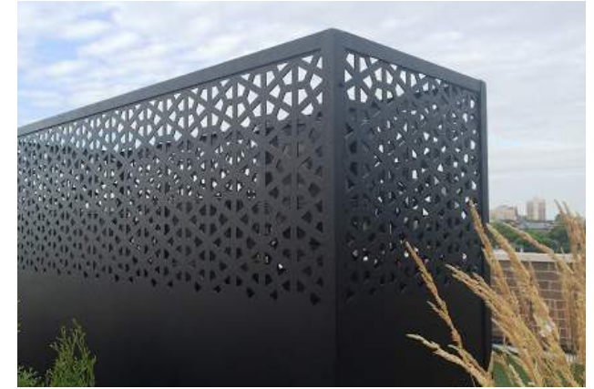
Metal Screening Hiding Mechanical/Utility Equipment
