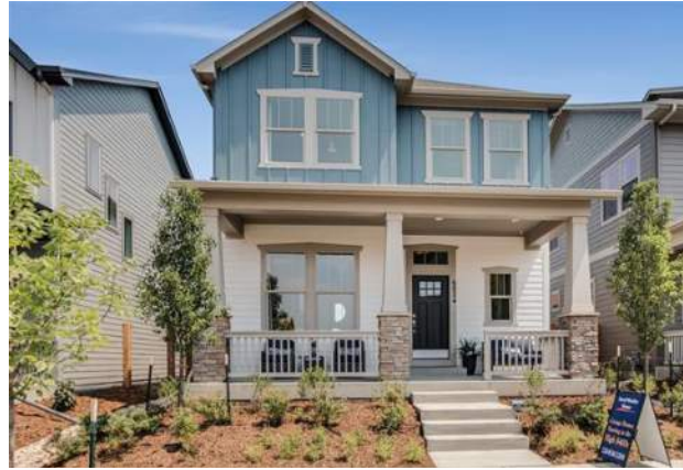
Entry Porches Facing Street
